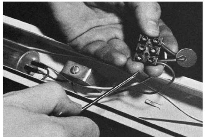
**SINGLE PHASE SURGE SUPPRESSOR CONNECTED ACROSS THE SUPPLY TERMINALS OF A FLUORESCENT LIGHTING FITTING.**
