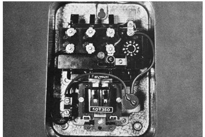
**SINGE PHASE SURGE SUPPRESSOR CONNECTED ACROSS CONTACTOR COIL TERMINALS.**
